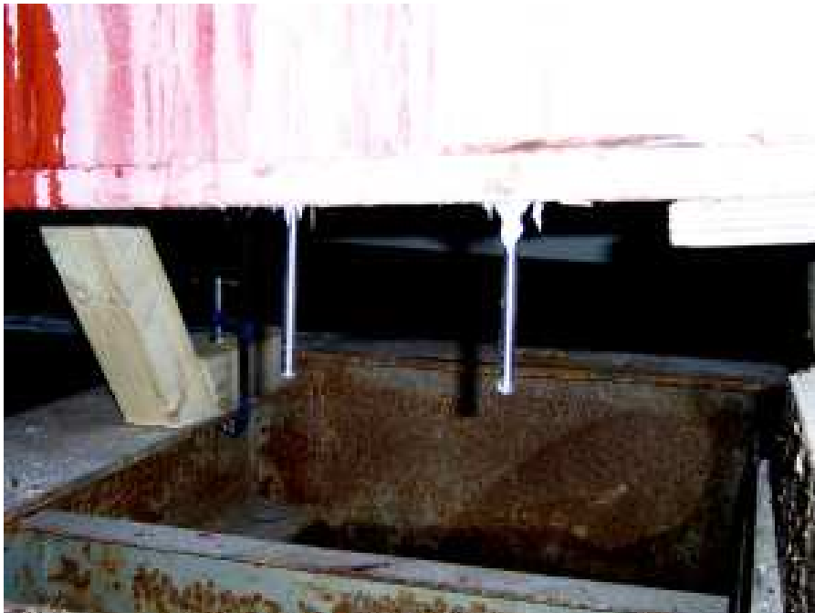
inserting a bolt through the keel from down to up
