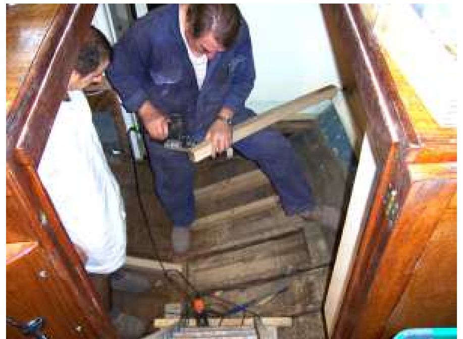
cutting a rib to fit
