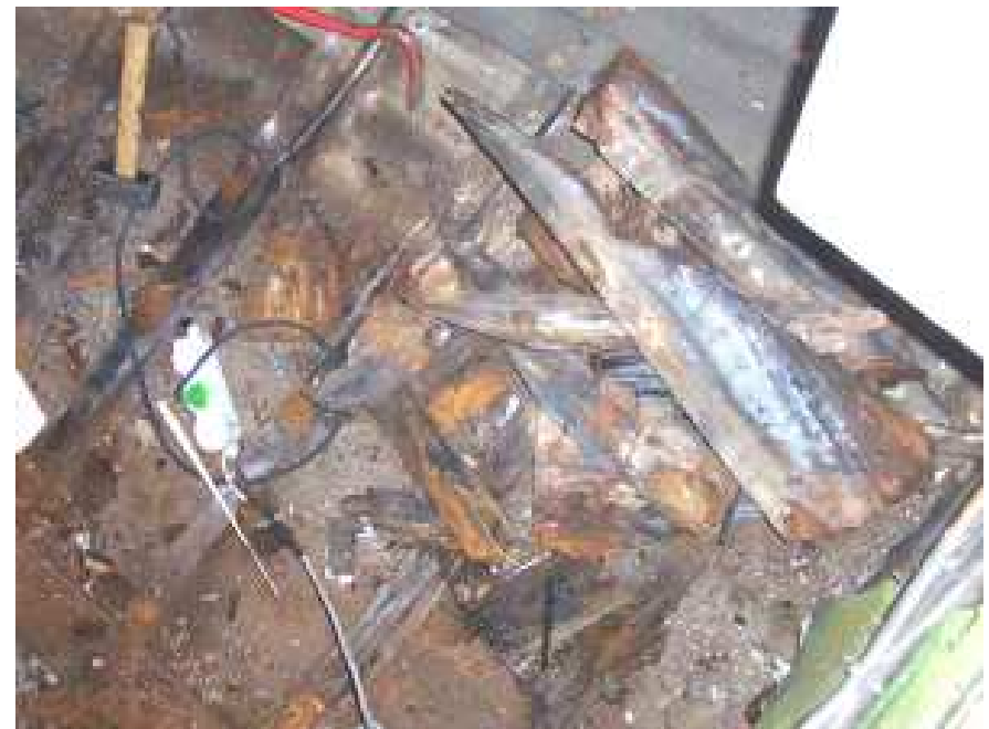
cut out rot pieces
