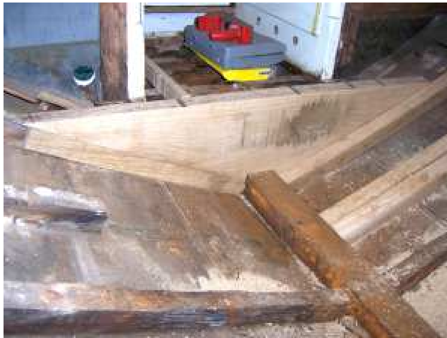
first floor (triangle piece) sitting on new ribs
