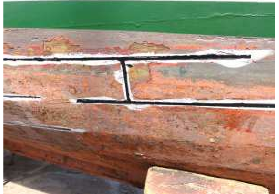
sealing with poleuretlan rubber
