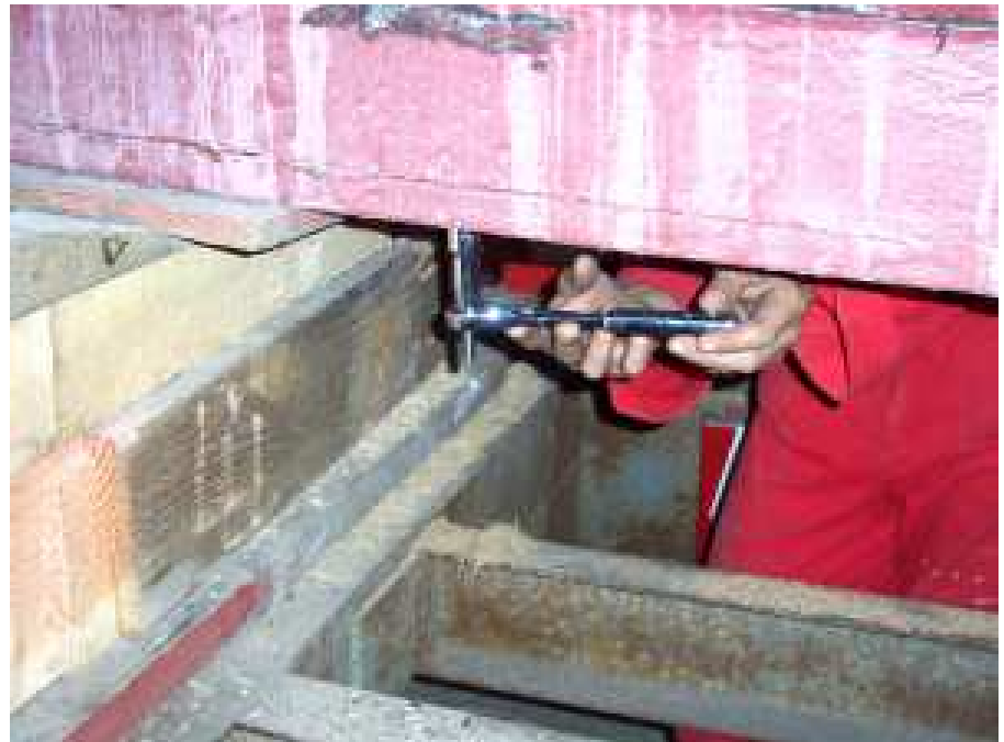
fastening the bolt, one man outside, one man inside
