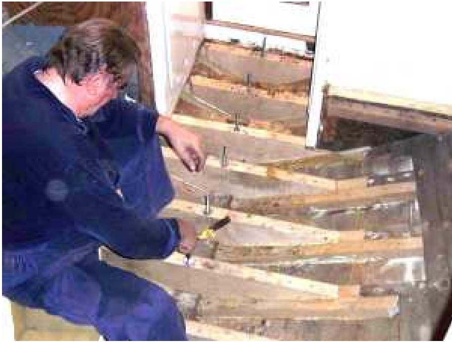
fasten with bolts through the keel
