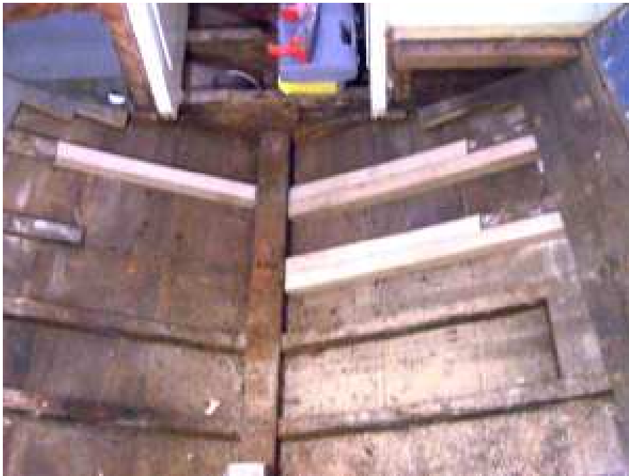
first three new ribs, two of them sistered
