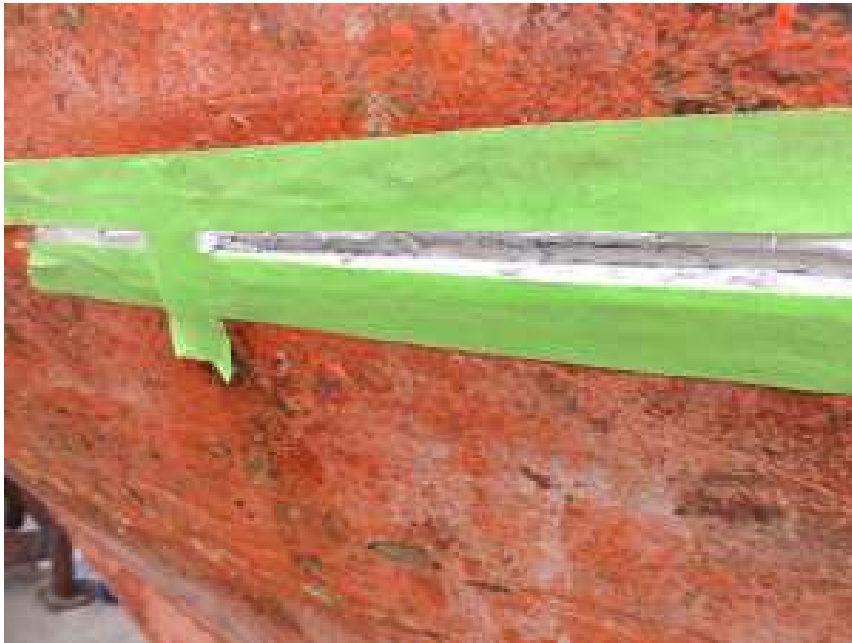
taping after caulking
