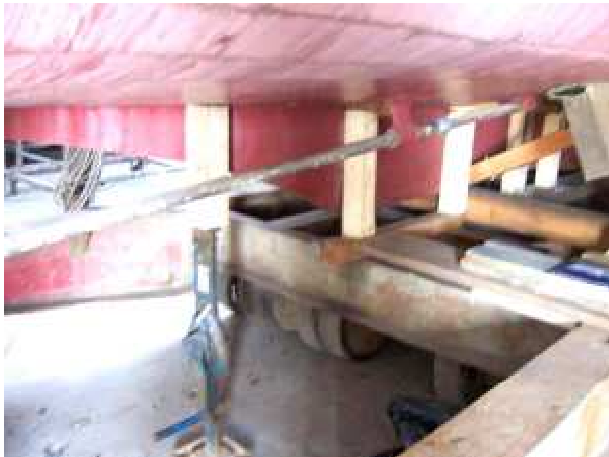
stabilize garboard (very first plank)
