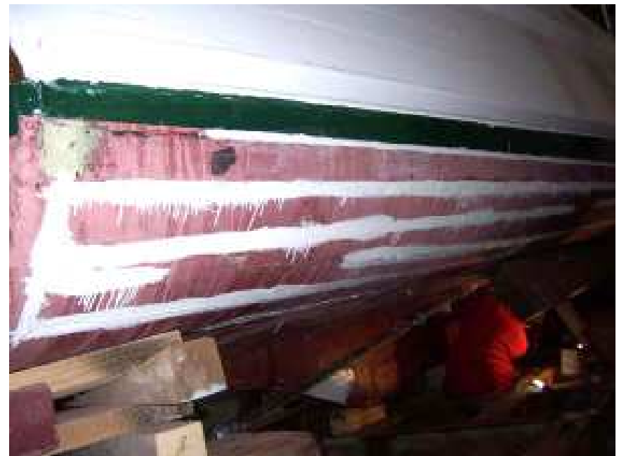
breaks caulked under the waterline
